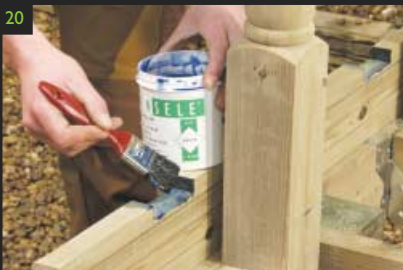
20 After carefully marking the boards notch out positions for the posts and treat with End-grain.
