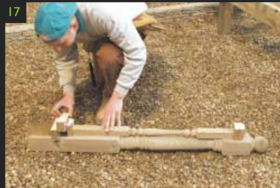
17 Calculate the height of the handrail by placing all the components on the newel post. Mark the height of the top of the joist.
